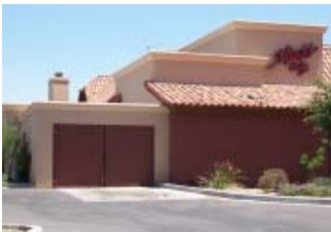
8.6 An example of a trash container enclosure that is architecturally compatible with the primary structure.
