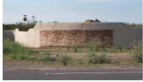
7.5 Example of preferred finish on perimeter fence.
